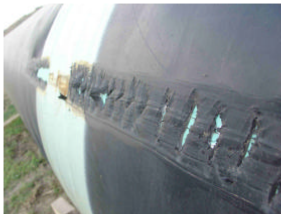
9 th October 2004, Pipeline laid by 18/19 th Districts, Rushtavi City
