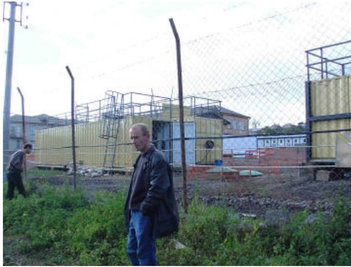
Mr Tavartkiladze stands at the edge of his land, next to BTC Co generators. The Mission measured the noise level at the spot above to average ninety db (10 th Oct 2004)
